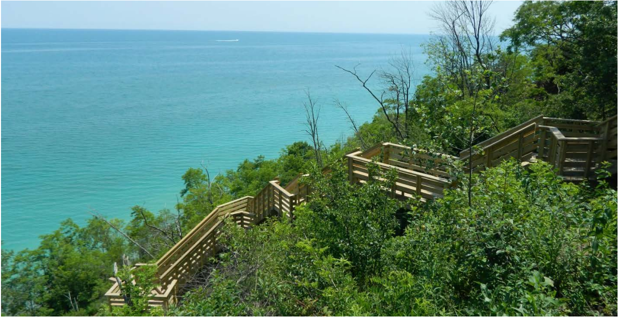
Partially Completed Stairway at Virmond County Park
