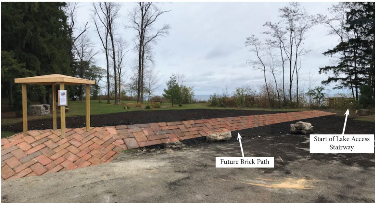
Location of Future Brick Path Leading to Lake Access Stairway
