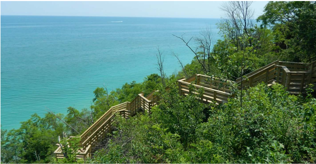
Partially Completed Stairway at Virmond County Park
