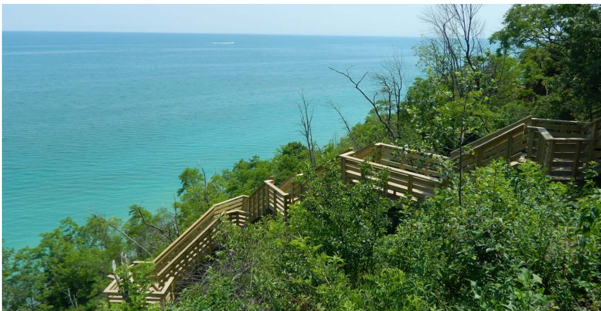
Partially Completed Stairway at Virmond County Park
