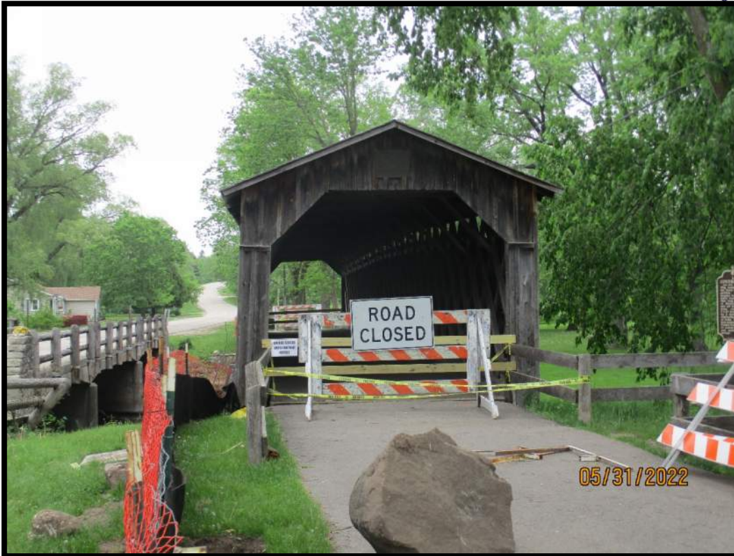
Figure 1: Top of structure looking North
