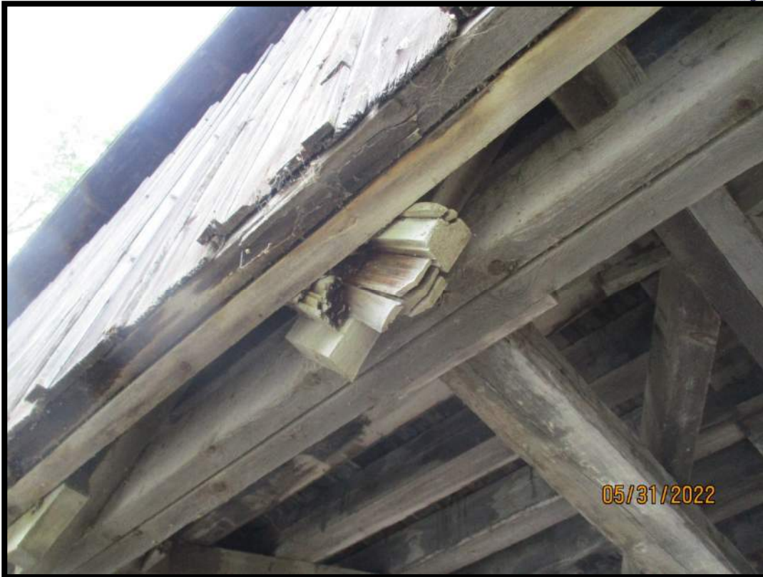
Figure 15: Truss Bottom Chord – Split in outer lamination
