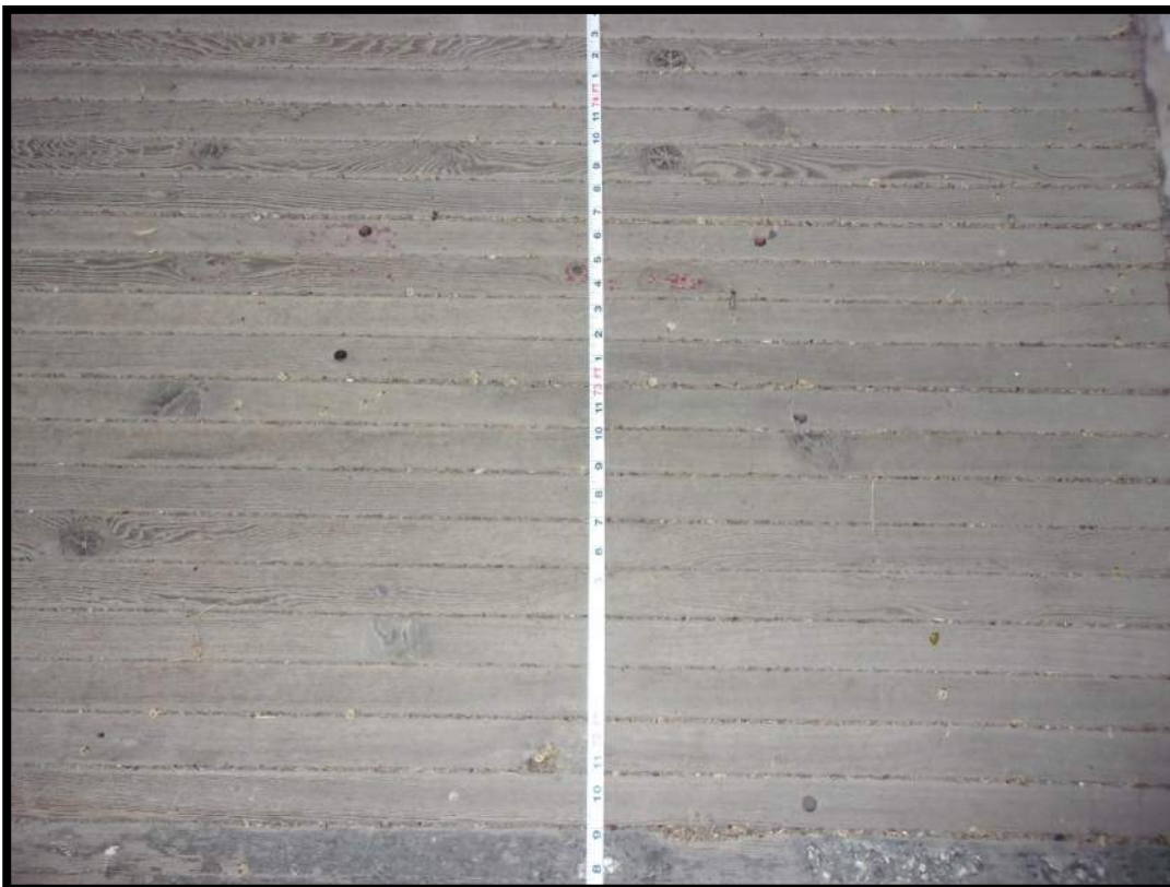
Figure 4: Typical timber deck surface
