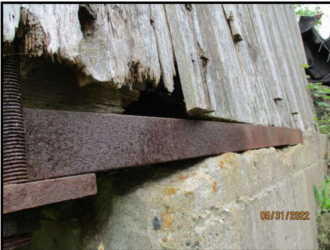
Figure 8: Truss Bearing at Abutment – SW Corner – Repaired with steel
