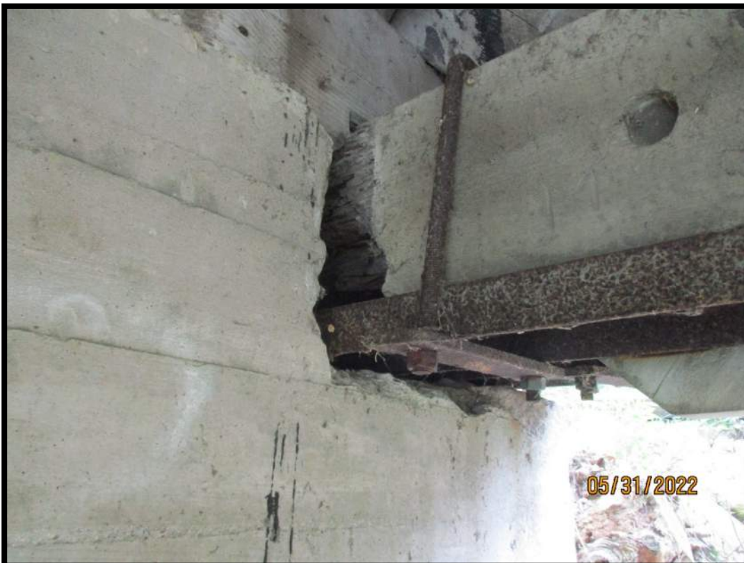
Figure 6: Truss Bearing at Abutment – SW Corner – Repaired with steel
