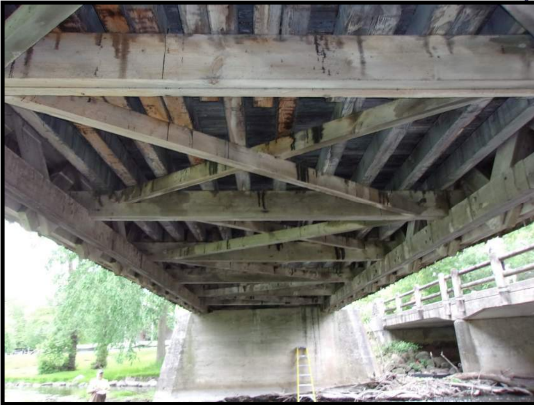
Figure 29: Stringer and Floor Beam Layout
