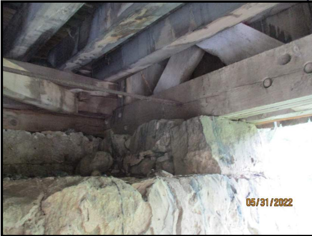
Figure 21: Truss Bearing at Abutment – NE Corner – No issues noted
