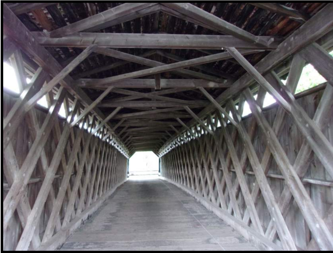
Figure 3: Inside of Structure
