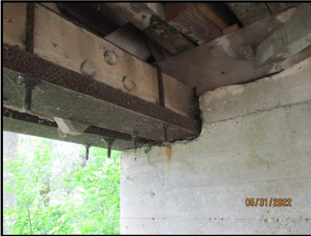
Figure 5: Truss Bearing at Abutment - SE – Repaired with steel
