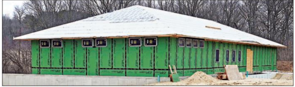
CONSTRUCTION OF A $374,000 multipurpose building at Hawthorne Hills Park is underway. It will house everything from an equipment storage area to bathrooms, showers and a kitchen. Photo by Sami Arendt
