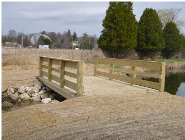
Wooden Bridge with Railings. Source, MeeKwon County Park
