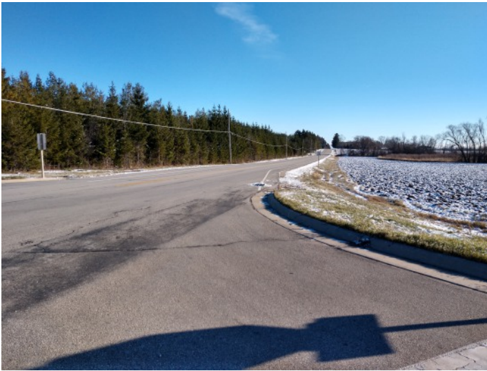
Northbound Granville Road looking east on CTH C/Pioneer Road
