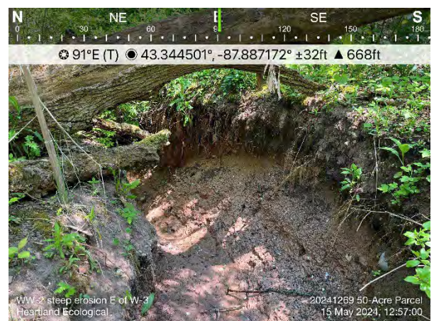
Photo #78 WW-2 steep erosion east of W-3
