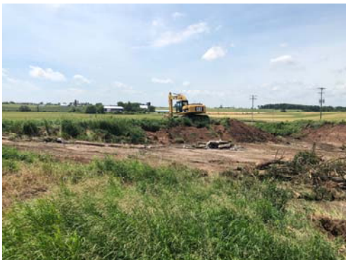
Manure Pit Abandonment project closed in 2024 on Hwy D in Belgium
