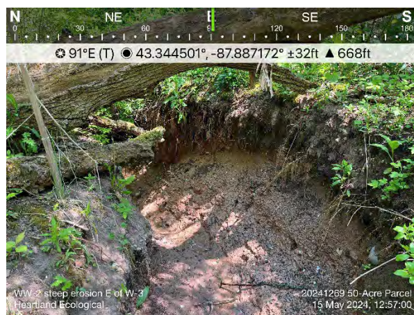
Photo #78 WW-2 steep erosion east of W-3
