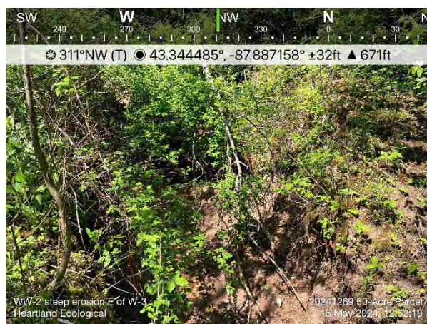
Photo #77 WW-2 steep erosion east of W-3
