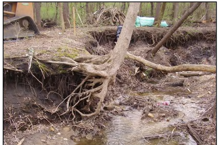
Before: Signature site with 9 foot severely eroded banks
