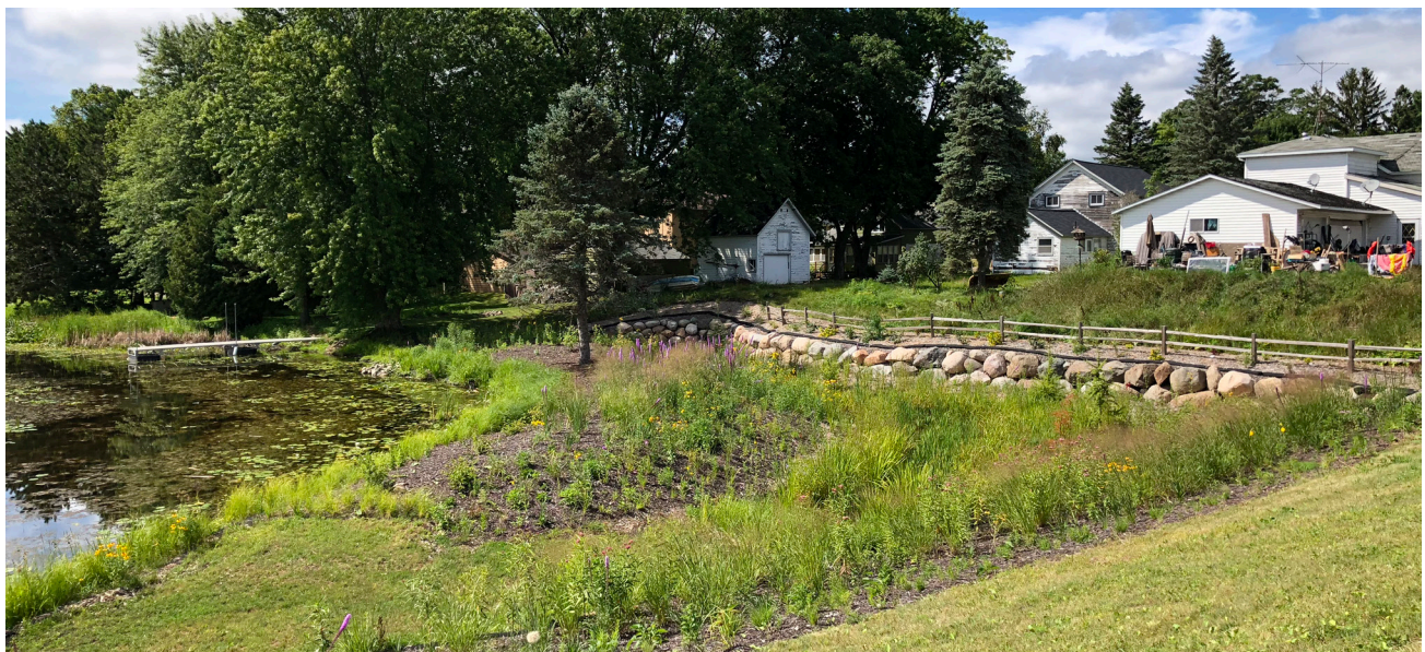
Library Lake, WI - Green Infrastructure Stormwater Management
