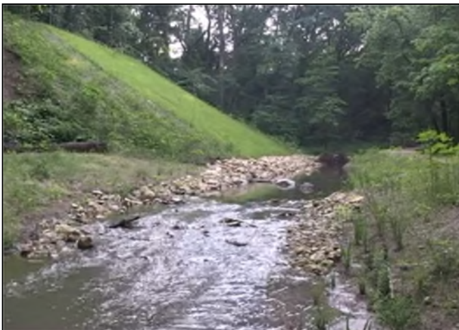
After Construction grade control, toe stabilization, and bluff bioengineering for the depicted above. Dead Dog Creek is a steep-sloped tributary to Lake Michigan.
