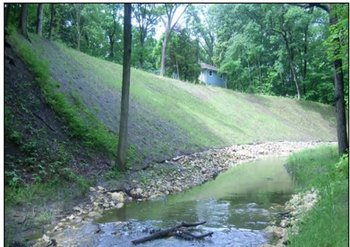
After Construction grade control, toe stabilization, and bluff bioengineering for the depicted above. Dead Dog Creek is a steep-sloped tributary to Lake Michigan.
